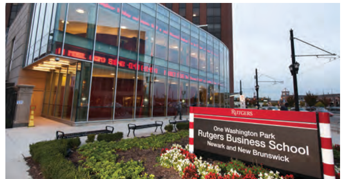
Rutgers Business School, Newark: The Engine Room
